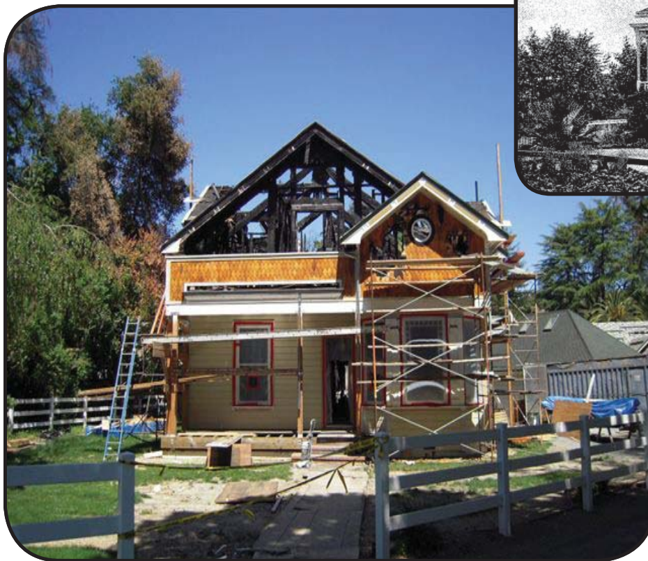
Historical home under renovation.
